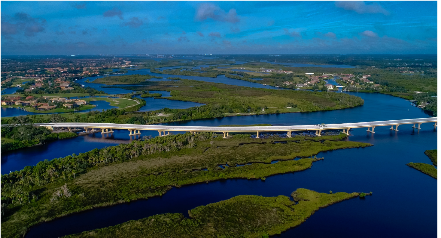
About 12,000 vehicles a day travel the Ft. Hamer Bridge which opened in October, 2017.
